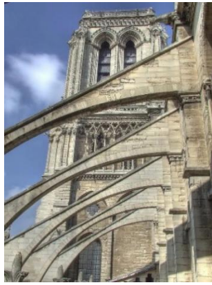
Figure 2. Flying Buttress
