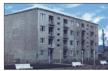
4-story apartment building with R/C monolithic load-bearing walls
