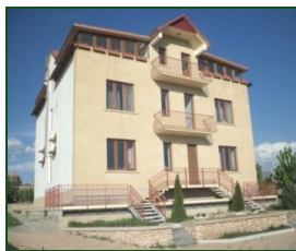
Single family house with stone, load-bearing walls
