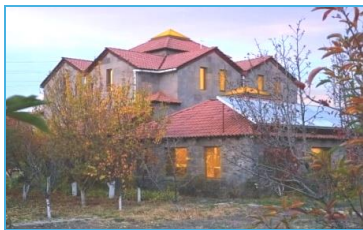
Single family house with stone load-bearing walls
