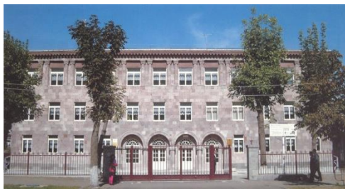
3-story stone school building retrofitted by base isolation
