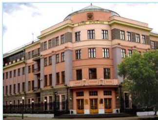
4-story existing stone bank building retrofitted by base isolation in the city of Irkutsk (Russia)
