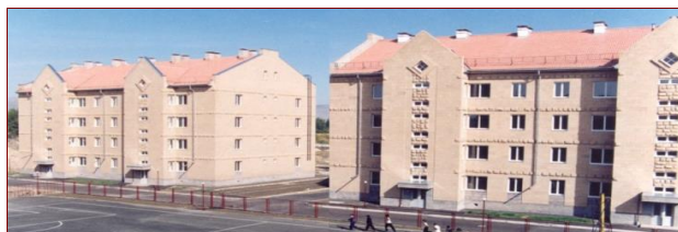
4-story apartment buildings with reinforced masonry load-bearing walls
