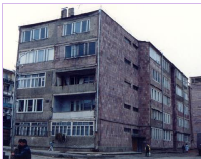
5-story stone apartment building retrofitted by base isolation
