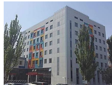
9-story R/C frame hematology center hospital building retrofitted by base isolation
