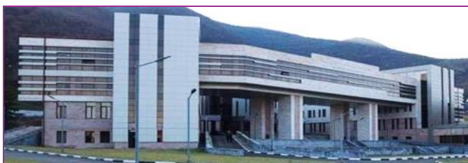
4-story Hospital R/C frame building with shear walls and asymmetric plan
